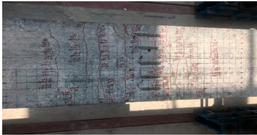
Figure 10. Formation and distribution of cracks in specimen 2: (a) Schematic view of cracks; (b) actual view of cracks.
