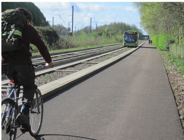
Fig. 1 The Cambridgeshire Guided Busway
