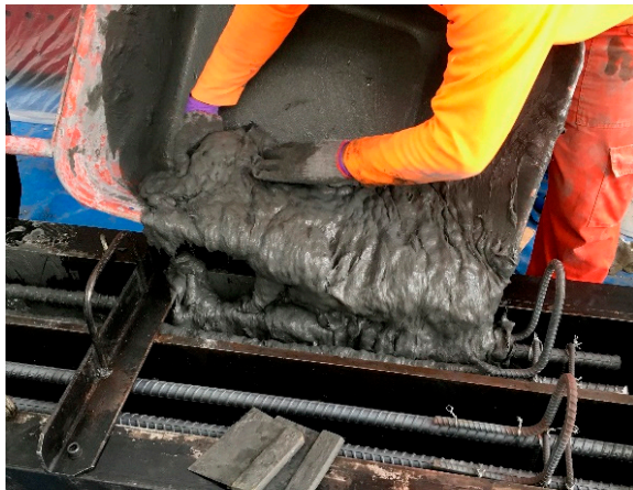
(c) Casting of the UHPC beams with PVA fibers
