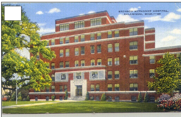
Fig. 1B. Bronson Methodist Hospital 1949 [Source: Local History collection, Kalamazoo Public Library, Michigan].
