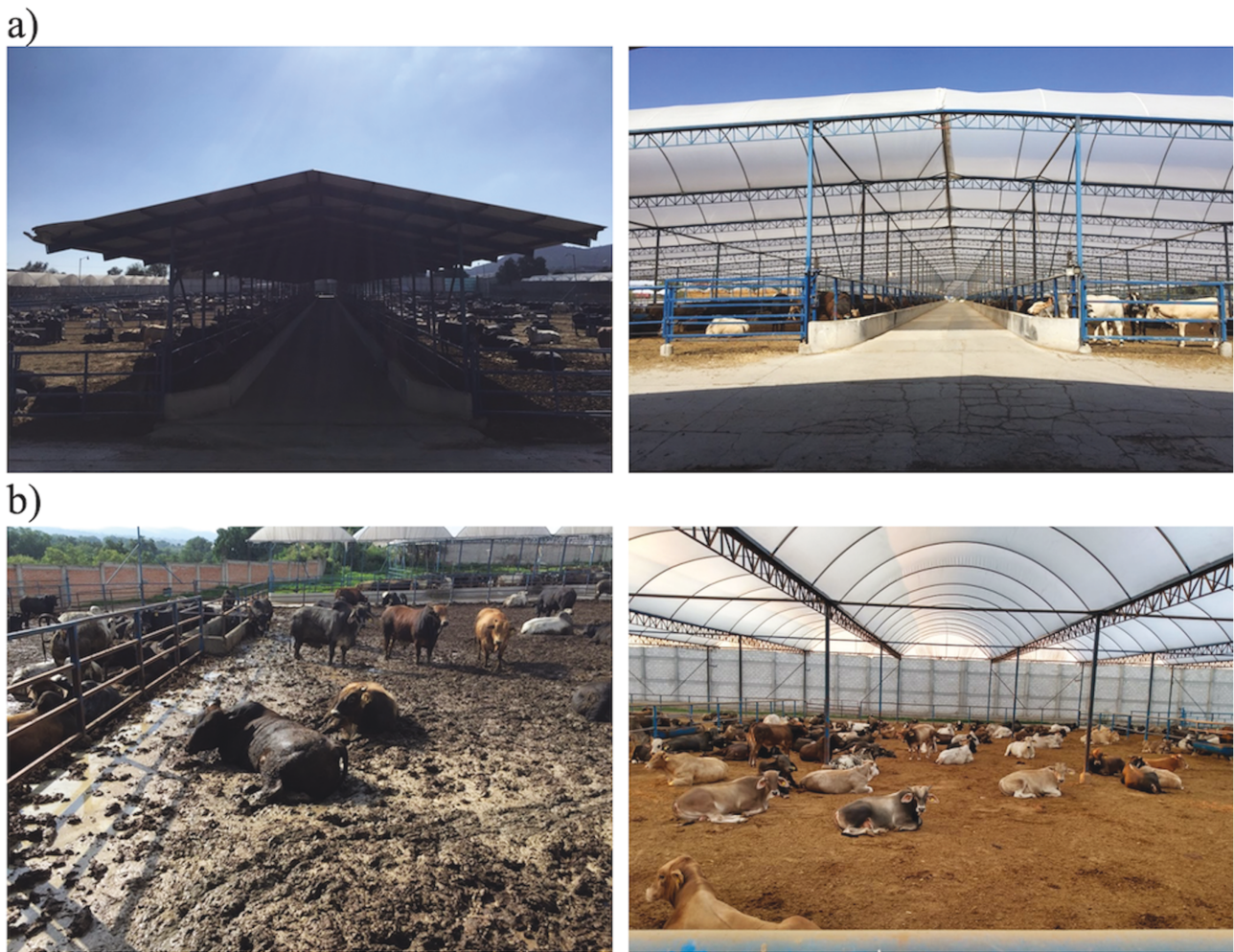
Figure 1. (a) General view of the design of pens without and with the greenhouse roof. (b) General view of the conditions of the pens without and with the greenhouse roof during the rainy season (June to September). Pens with greenhouse roofs are covered, and they stay dry even in the rainy season. Pens without the greenhouse roof only have covered the bunk area and are muddy during the rainy season, demanding frequent cleaning.
