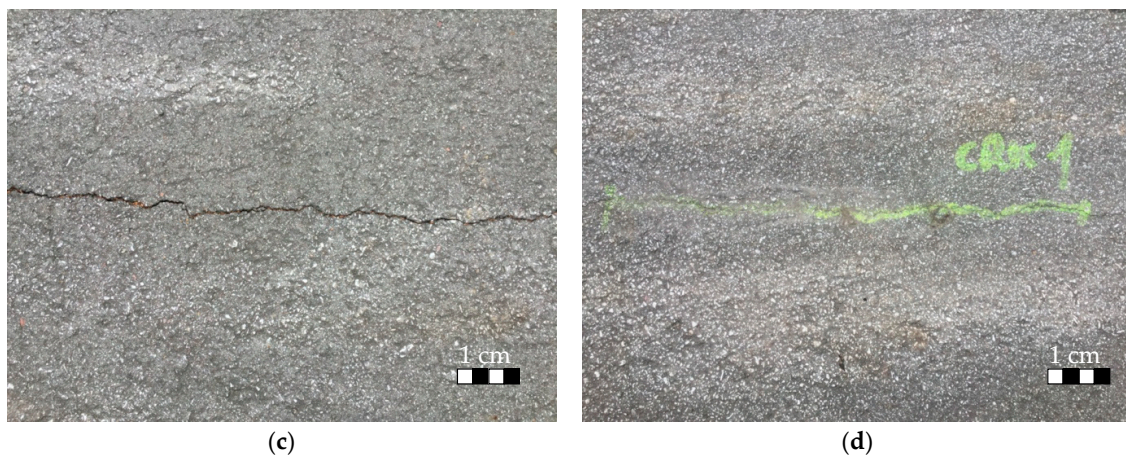
Figure 13. (a) Illustration of real-scale test section microwave-assisted asphalt pavement repair (cores were taken from nearby locations), core from the pavement before MW treatment; (b) Core from the pavement treated with MW; (c) Cracked pavement before MW repair (crack width ca. 5 mm, crack depth–12 cm, full pavement depth), (d) Cracked pavement after MW repair.
