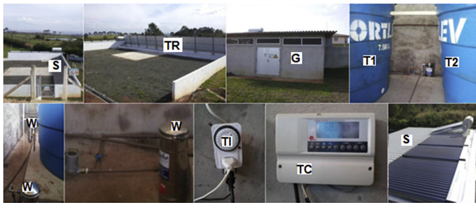
Figure 1. Evaporation process of water obtained from the washing of pesticide containers used for DNA collection in this study. S: sanitary sink; TR: tractor spray washing trough; SH: shed where the two tanks (T1 and T2) are located; T1: tank 1; T2: tank 2; W: water filters; TI: timer for controlling the flow of water; TC: solar heating temperature control panel; and So: solar heating system.
