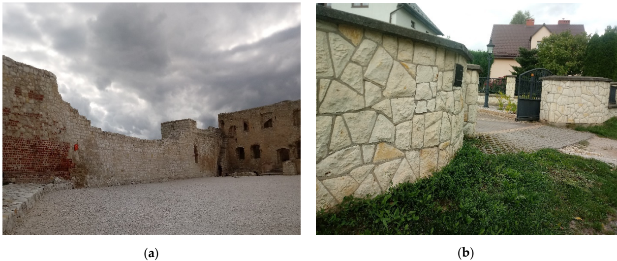
Figure 3. (a) The walls of the Castle in Kazimierz Dolny on the River Vistula, made of opoka rock. 14th century; (b) Contemporary use made of opoka rocks from the Bochothnica region (author's own elaboration).
