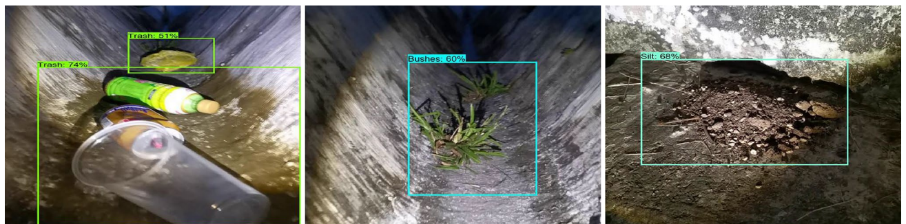
Figure 18. Real time drain inspection field test (night).
