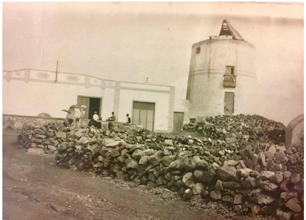
Figure 14. Flour mill of SB (1870), erected by Baltasar Fermín and acquired by José María Gil in 1919, today declared a Site of Cultural Interest (BIC).
