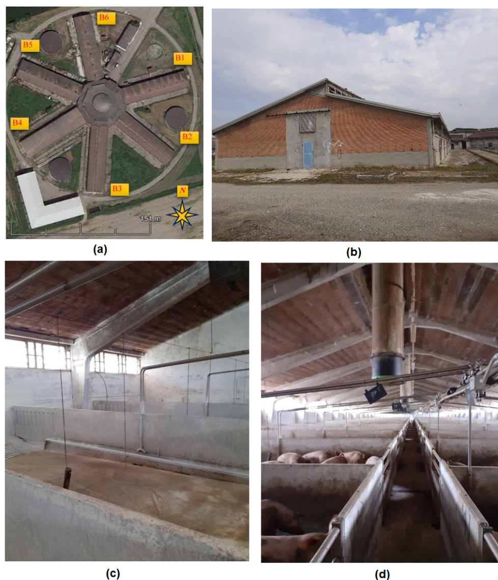
Figure 1. The case study building: (a) aerial view of the farm; (b) external view of building B3 (naturally ventilated); (c) internal view of building B3 (naturally ventilated); (d) internal view of the building B5 (mechanically ventilated).
