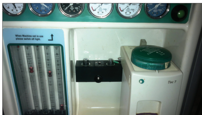
Figure 1: Needle causing the leak
