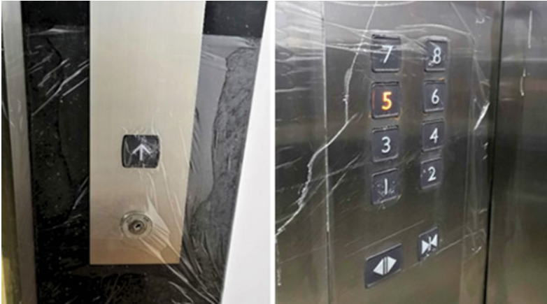
Fig. 5.67 While considering protection measures, it is more than just the generalities but also details of certain aspects that require further attention. For instance, here we see examples of adhesive plastic wrap covering the area where we touch the most on a regular basis. They are disinfected regularly and are replaceable easily. Doing this is a simple measure but also effective not to damage the buttons due to regular disinfection procedures. Source Ali Cheshmehzangi
