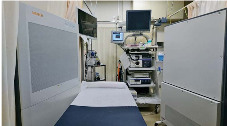
▶ Fig. 1 Portable partitions with high-efficiency particulate air (HEPA) filters were placed in the endoscopy unit.
