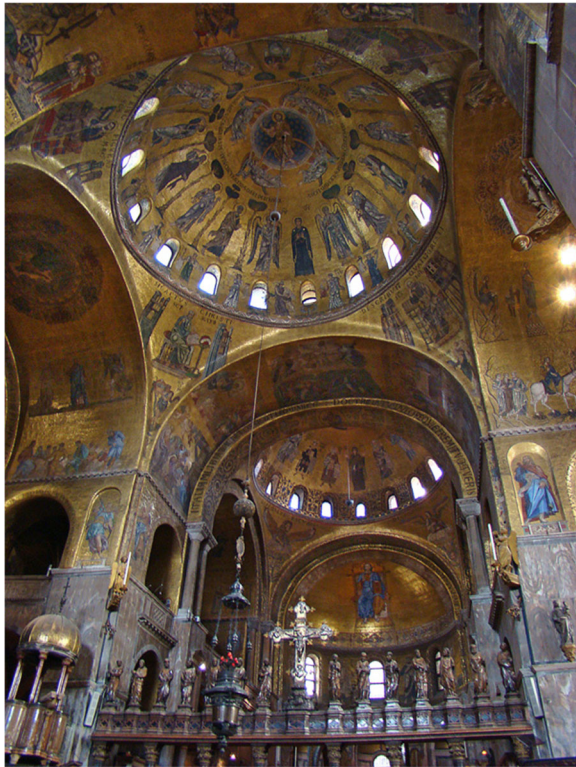
Fig. 1. The spandrels of San Marco. The structures that support the arches of the San Marco basilica in Venice are notable for the pictures that decorate them; however, the original role of these structures (spandrels) has nothing to do with the images they carry
