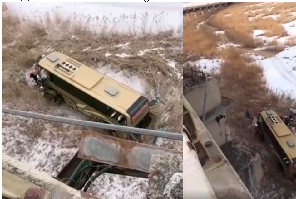
(b) The bus crashed into a guardrail and fell under the bridge
