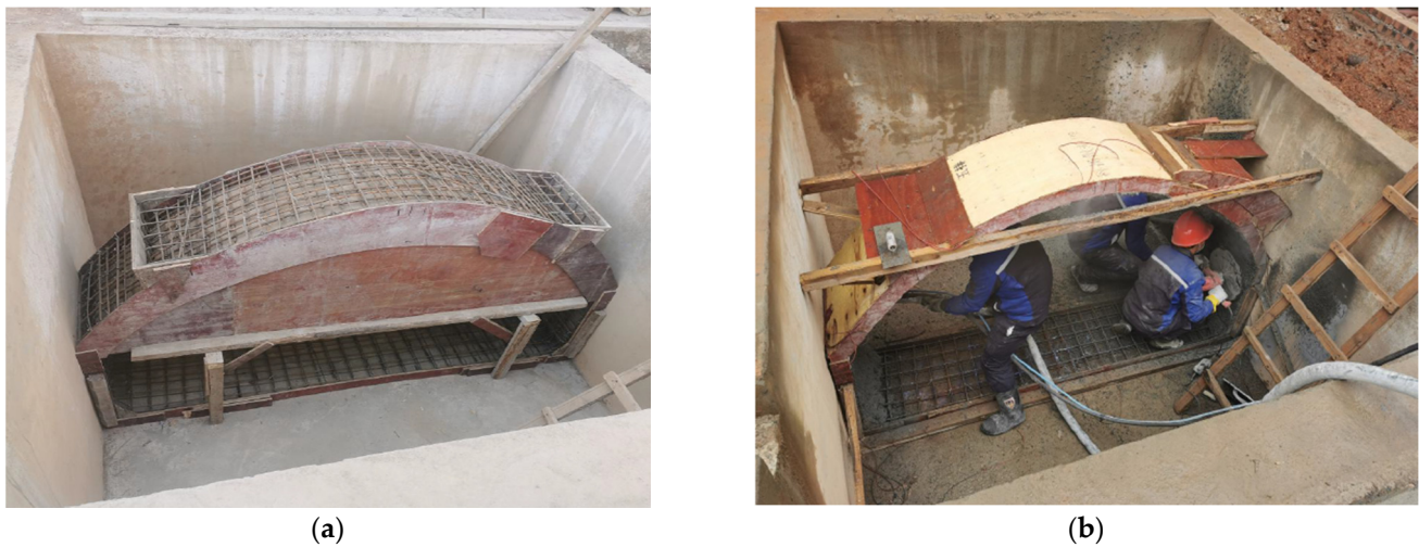
Figure 3. Test model. (a) assembling reinforcement; (b) spraying concrete.
