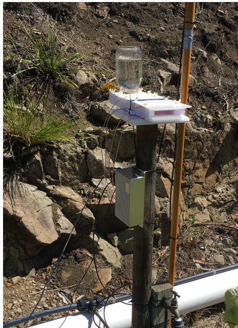
Figure 5. Feeder station equipped with the presented system.
