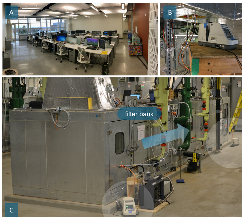
Figure 2. UFP monitoring for the office and its air handling unit with a diffusion charger sensor array. (a) Room air diffusion charger sampling location in the living laboratory office. (b) Outdoor air intake diffusion charger sampling location. (c) Diffusion charger sampling locations for the supply air upstream and downstream of the HVAC filter bank. An arrow is included to show the airflow direction for the supply air through the air handling unit.
