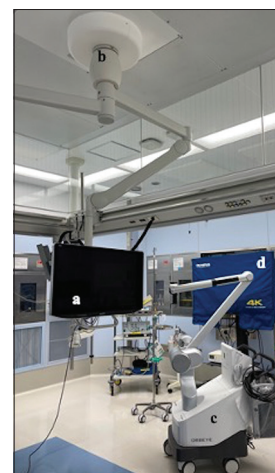
Figure 1: Set-up of 31-inch movable 4K 3D monitor. The 31-inch movable 4K 3D monitor installed in the Maquet Moduevo ceiling supply unit. The monitor can be moved in response to the operative site. (a) A 31-inch movable 4K 3D monitor (b) Maquet Moduevo ceiling supply unit c: ORBEYE™ main body d: A 55-inch 4K 3D monitor (covered by blue cloth).
