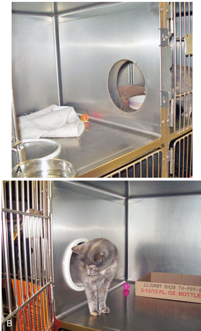
FIGURE 46-23 A and B, Conversion of existing cages into condo-style units. A hole is cut through the walls of adjacent cages and a section of polyvinylchloride (PVC) pipe with corresponding rims are used to create a safe portal for passage between the cages.
