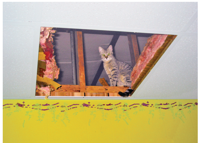
FIGURE 46-31 A solid-surface ceiling is essential in free-range housing rooms to prevent the escape of cats into the rafters. Once in the ceiling, cats may be difficult to recover, and injury and/or damage to the facilities may result. (From Griffin B, Hume KR: Recognition and management of stress in housed cats . In August JR, editor: Consultations in feline internal medicine , vol 5, St Louis, 2006, Elsevier, p 717.)
