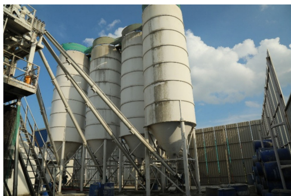
Figure 2. Storage of cement, fly ash, and GGBS in silos.
