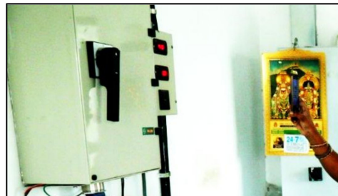
Figure 4. Recording the power meter reading during the mixing operation.
