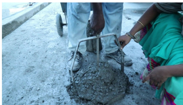
Figure 8. Measuring the slump value.
