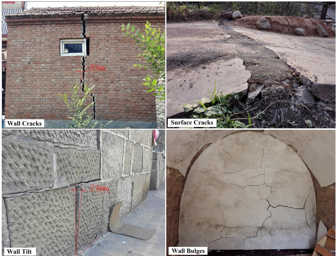
**Fig 2. Examples of damage to village buildings.** (A) Wall cracks. (B) Surface cracks. (C) Wall tilt. (D) Wall bulges.
