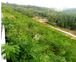
Figure 22. Growing green plants on the slope.
