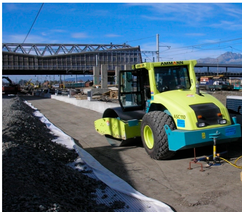
Figure 9. Static load tests on the compacted layer.
