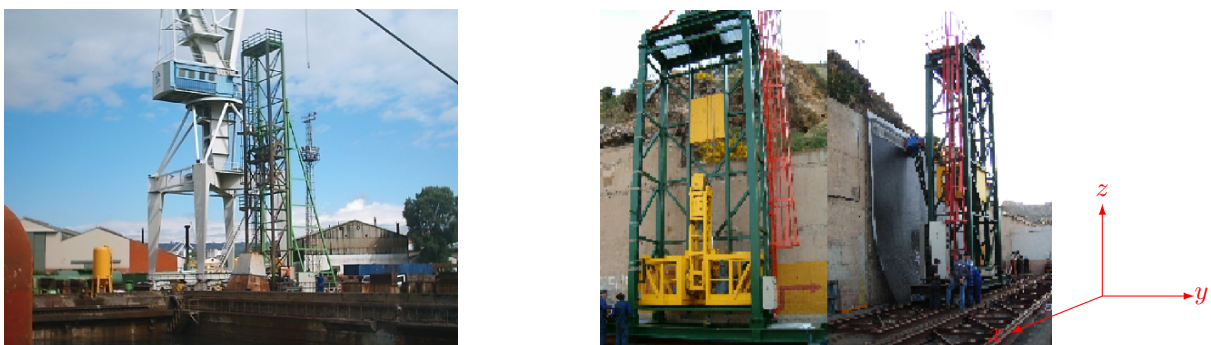
Figure 4. Primary Structure Vertical Towers.
