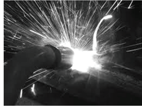
FIGURE 2: Opening for electric arc welding activity.
