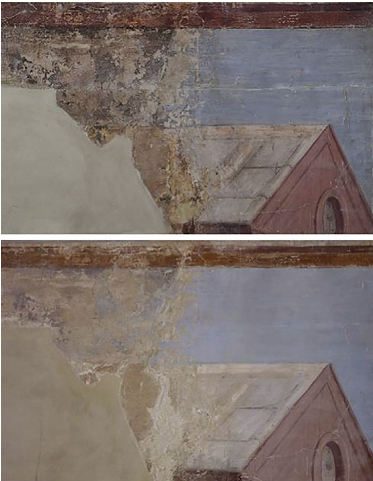
FIGURE 15.6 Effect of biocleaning with Pseudomonas stutzeri bacterial strain on the Stories of the Holy Fathers fresco before (top) and after (bottom) treatment [99].
