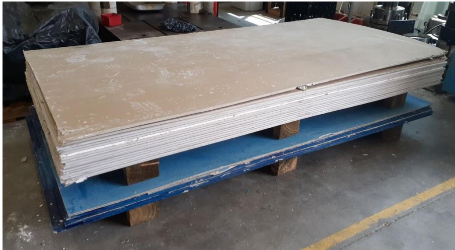
Figure 4. Infill panels: (top) gypsum plasterboards, (bottom) cement- or blue-boards.
