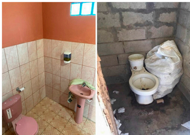
FIGURE 1. Characteristics of bathrooms with flushing toilets (left panel) and latrine cabins (right panel) in Atahualpa. Differences in sanitation are evident between these facilities. Bathrooms have an incorporated piped water sink and most often have disinfecting fluids for handwashing. By contrast, latrines do not have incorporated pipe water sinks and are under poor hygienic conditions, toilet papers are accumulated on open bags or all over the floor, and there is macroscopic evidence of fecal material in some of their inner walls. This figure appears in color at www.ajtmh.org .
