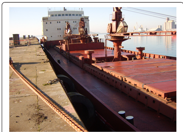
Figure 1 Bulk carrier where the poisoning occurred.
