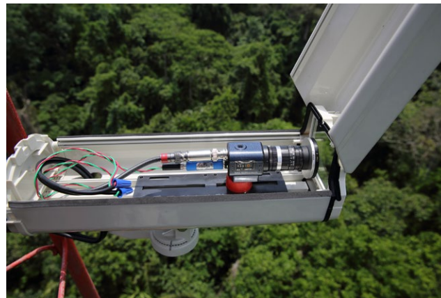
FIGURE 1 A surveillance camera mounted on one of the towers used in the video network for lightning monitoring. A 3.0 neutral density filter is attached to the front of the camera, and both the power supply and video feed cables are fitted with in-line surge protection. The complete setup is protected within a metal box, which is open for the photograph
