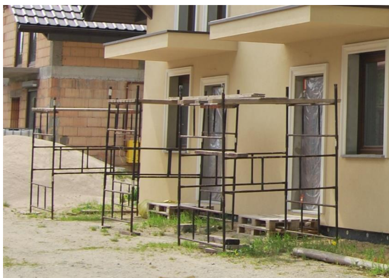
Figure 1. The example of the Warsaw-type scaffolding (author's archive).
