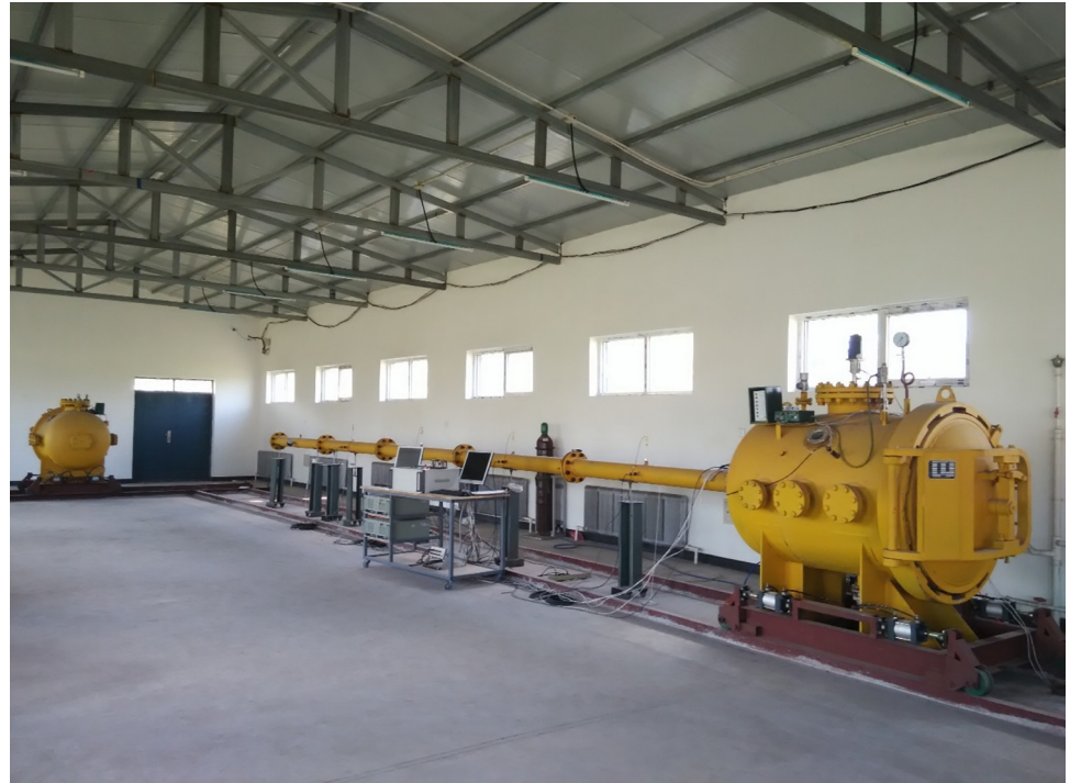
Fig 2. The testing platform of the tube gas explosion: Experimental setup.
