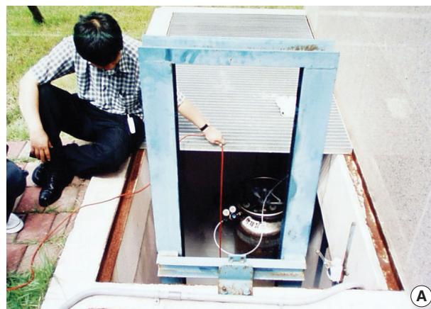
Fig. 1. The accident site in the underground dry area showed a LN 2 cylinder and a Dewar-flask that were linked to a copper tube in front of two O 2 tanks in a corner.
