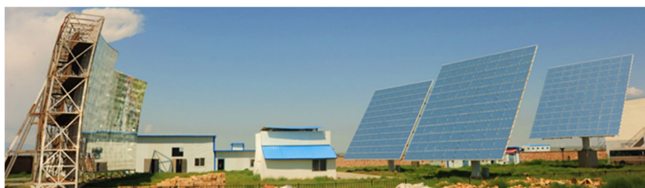
Fig. 6 Pilot-scale demonstration plant of SCWG system driven by concentrated solar energy, reprinted from [34]
