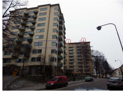
Figure 3. View to the low exposure apartment (rectangle). Mobile phone base station antennas are visible on the neighboring building (circled); the highest RF exposure level was on the balcony, which had the line of sight to both of the antennas. However due to the elevation difference, the balcony had highest electric field only 0.75 \text{ V m}^{-1} ; based on spot measurements maximum readings over 1-min period; base station antennas' sector include the investigated building. Rectangle, low exposure apartment; circle, neighboring building. RF, radiofrequency.
