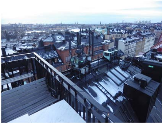
Figure 2. A view from the high exposure apartment's balcony, a set of mobile phone base station antennas are 6 m away from the fence; this was the highest radiation area, with the RF exposure topping at 6 \text{ V m}^{-1} , even though the antennas sector was positioned away from the balcony. RF, radiofrequency.
