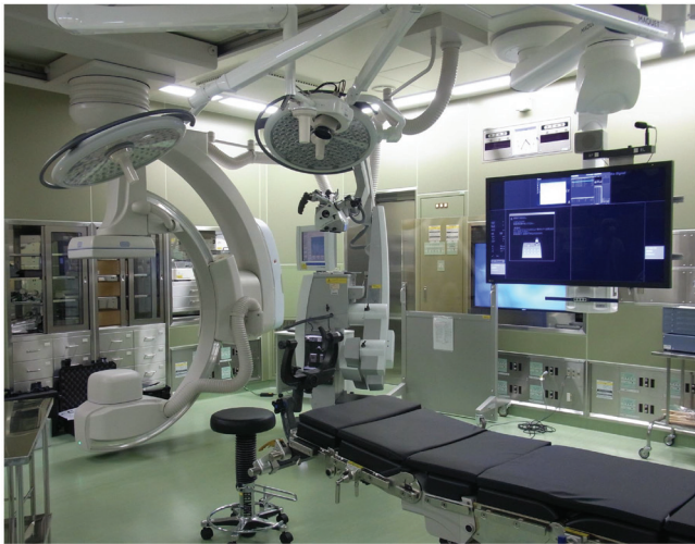
Fig. 4 Hybrid operating room at Hokkaido University Hospital, Sapporo, Japan. Single-plane neuroangiographic digital subtraction angiography units.
