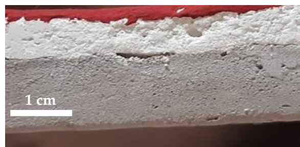
Figure 1. Stratigraphy of the specimens; from the bottom: concrete, plaster, painted layer.
