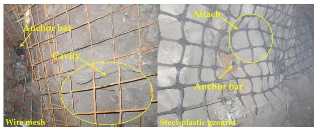
**Figure 17.** Comparison of the degree of fit of the mesh to the surrounding rock.
