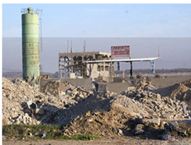
(a) Pile of demolition debris
