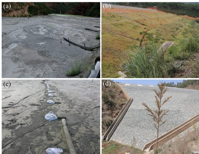
**Figure 1.** Engineering field of the tailings pond: (a) dry beach; (b) slope surface; (c) sampling points on dry beach surface; and (d) initial dam.
