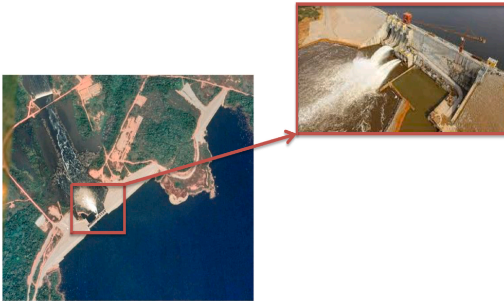
Fig. 1. Location of the Lom Pangar reservoir.
