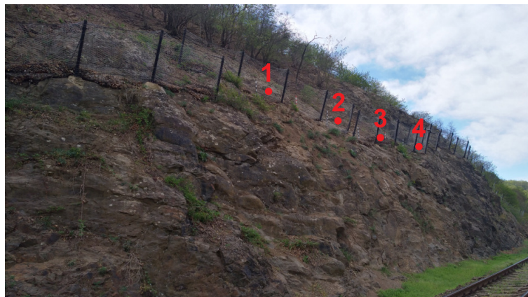
Figure 11. View of the installed protective fences above the railroad.
