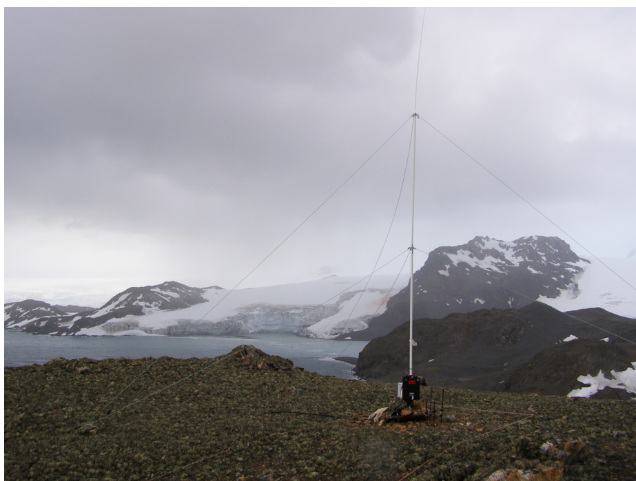
Figure 1. Antenna of the oblique ionosonde transmitter placed at the SAS.
