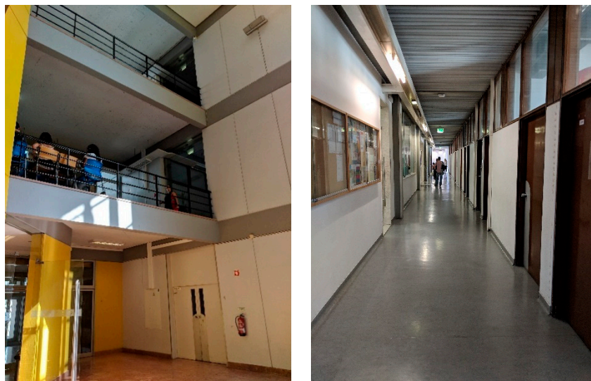
Figure 4. Signal propagation test locations: mezzanine (Left) and corridor (Right).
