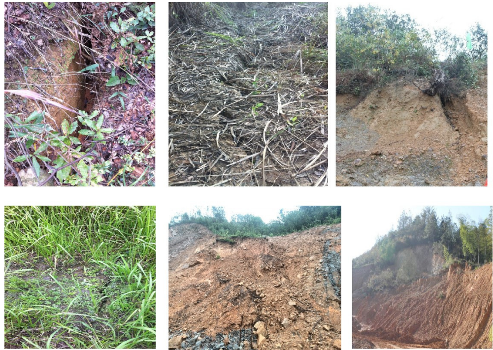
Figure 4. Cracks and deformation in the field.
