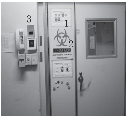
Fig. 15. Multiple signage. 1: Activated pathogens symbol, 2: Biohazard sign, 3: Lock pad (a security feature)
