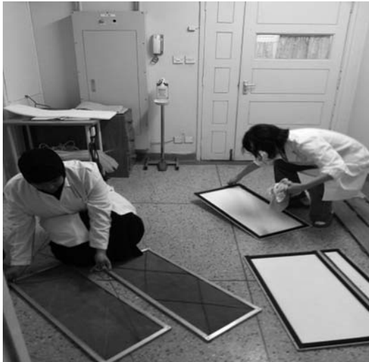
Fig. 7. Lab staff changing pre-filters
