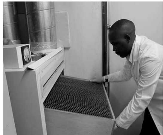
Fig. 10. Lab staff removing used-up intermediate filters
