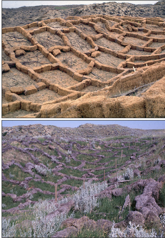
Fig. 5. Straw bale grid placed on the surface to act as a wind barrier (top) until vegetation is established (bottom).
