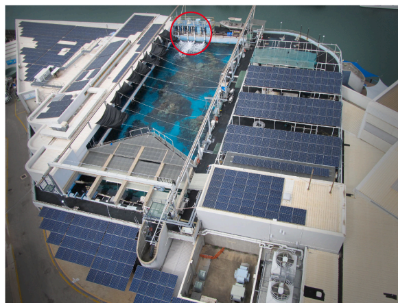
Fig. 2. ‘The Aquarium’ and specific site of the filtration system used for the study (circled in red) (photo credit: Queensland Fire and Rescue Service). (For interpretation of the references to colour in this figure legend, the reader is referred to the Web version of this article.)
